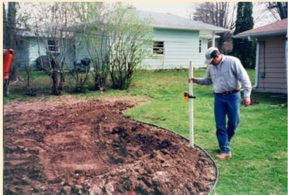
The rain garden is dug to 3 to 4 inches in depth with care to make the bottom as level as possible. With the lawn sloping gently upward to the house, the garden is positioned to trap water from a downspout.
